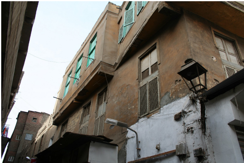
Fig. 12 Upper floor projection in the façade of an Ottoman house in Cairo. ©Hossam Mahdy
