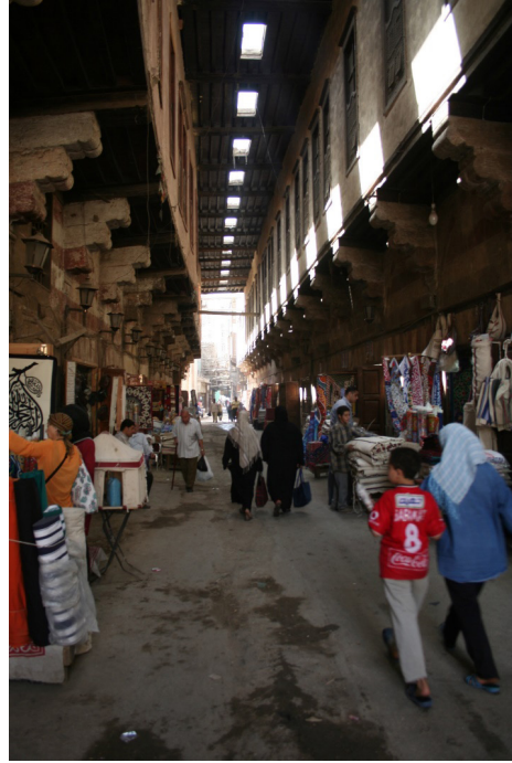
Fig. 2 Wooden shading structure with skylights, Qasabet Radwan, or Al-Khayamiyyah, Cairo. ©Hossam Mahdy
