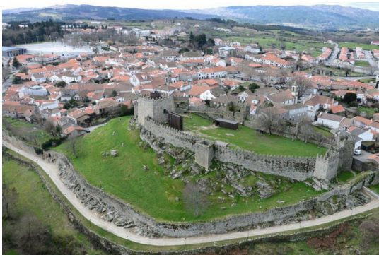
Fig. 34 Castle in Trancoso, Portugal, source: https://www.archdaily.com.br/br/01-189232/adequacao-do-patio-do-castelo-de-el-real-de-la-jara-slash-villegas-bueno-arquitectura?ad_medium=gallery , access August 2023
