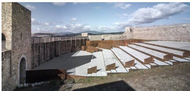
Fig. 36 Castle in Castello del real de la Jara, Spain, source: https://www.archdaily.com.br/br/01-189232/adequacao-do-patio-do-castelo-de-el-real-de-la-jara-slash-villegas-bueno-arquitectura?ad_medium=gallery , access August 2023
