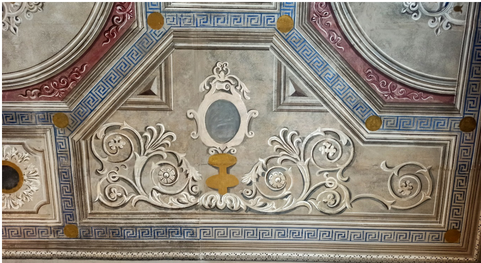
Fig. 6 Mansion of G. Modiano, painted ceiling decoration, after restoration
