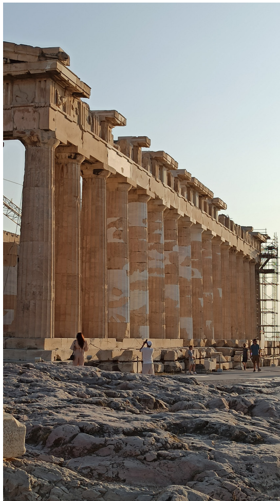
Fig. 12 Parthenon, north colonnade, after the restoration works of 2000 - 2010
