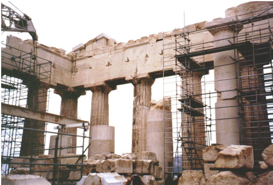
Fig. 11 Parthenon, pronaos columns, after the restoration works of 2001
