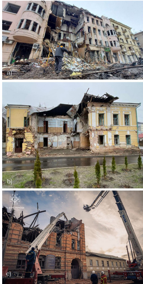
Fig. 8. a) 8 Svobody Street, D. Hrebynnyk/Souspilne, March 2022, b) 13 Poltavsky Shlyakh Street, (Paramonov, December 2022, c) 77 Goldbergivska Street, Main Directorate of the State Emergency Service of Ukraine in Kharkiv Oblast, November 2023
