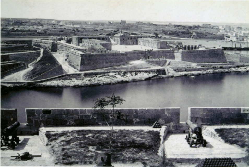
Fig. 8 View of Church of St Anthony of Padua in Fort Manoel, Manoel Island from the Valletta landfront [AoM consortium]
