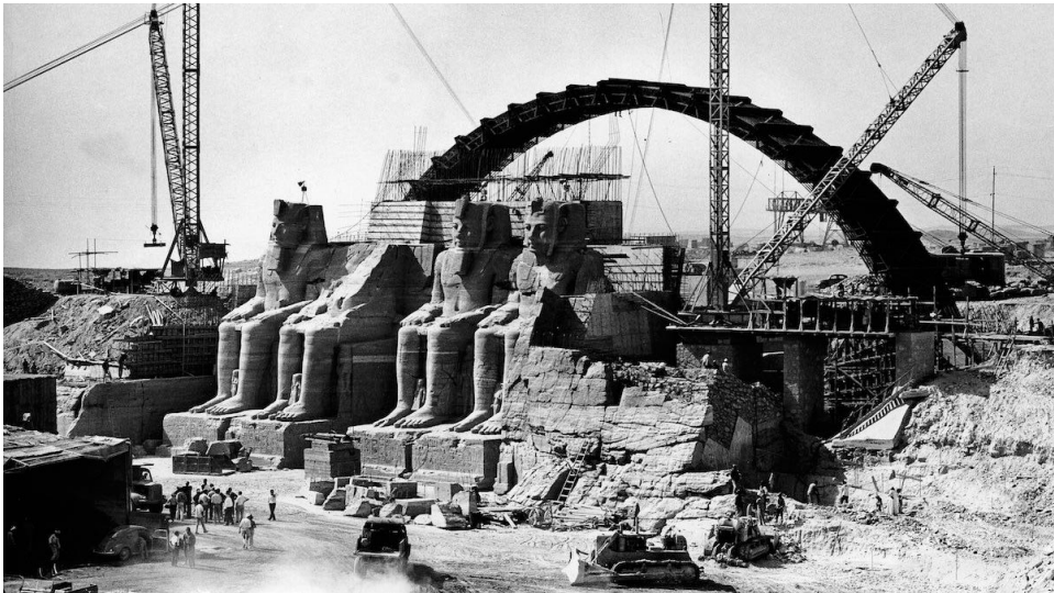
Fig. 2 During the move of Abu Simbel temple. https://www.tripsinegypt.com/wp-content/uploads/2018/12/Abu-Simbel-Temple-Relocation-Process-Step-by-Step-Trips-in-Egypt-1.jpg
