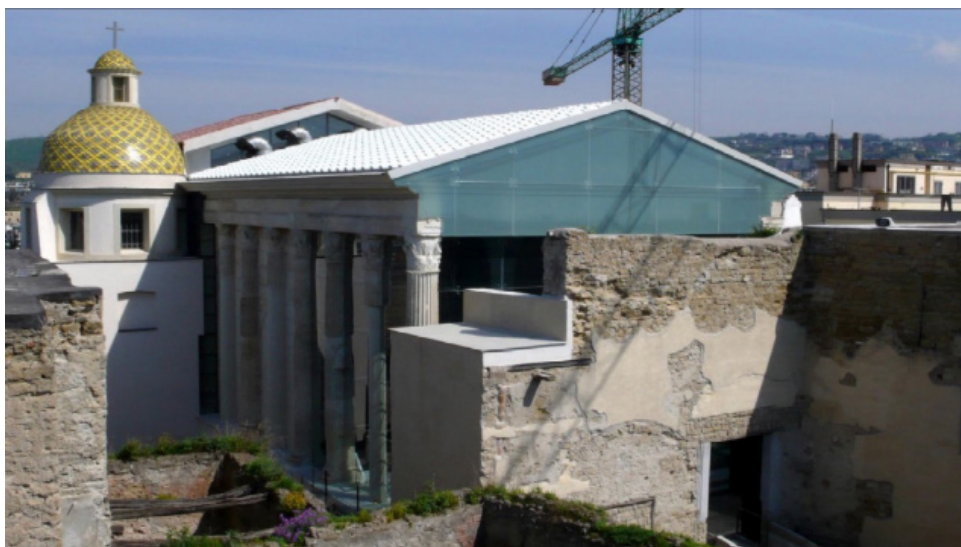
Fig. 11 View of Temple-Cathedral showing the external wall of the Baroque cathedral and the wall of the current Temple-Cathedral. [Source: Prof. L. Migliorati]
