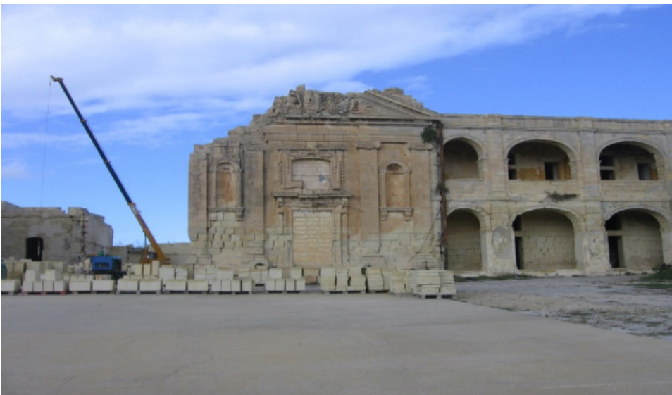
Fig. 9 Image of Church of St. Anthony of Padua after war damage [AoM consortium]
