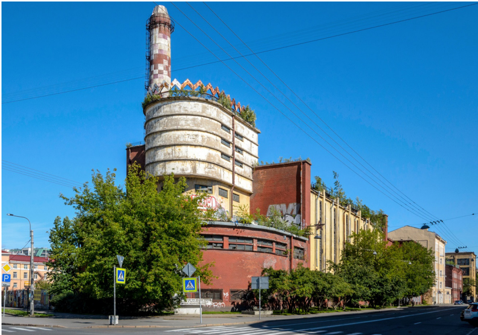
Fig. 5 Power Station of the Red-Banner Textile Factory, Petersburg, E. Mendelsohn, 1925-26 – due to the bad state of preservation excluded from the nomination (source: https://en.wikipedia.org/wiki/Red_Banner_Textile_Factory#/media/File:Power_Station_of_the_Red_Banner_Textile_Factory_SPB.jpg )
