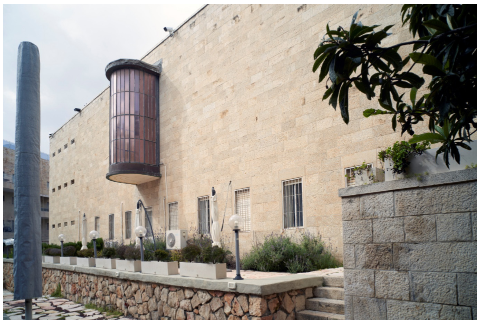
Fig. 4 The Schocken Library, Jerusalem, E. Mendelsohn, 1935-36 – different climate, different tradition, different building material (photo Jerzy Ilkosz, 2023)
