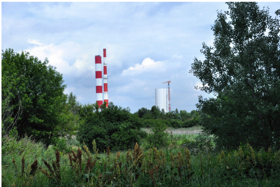
Fig. 11 Chimneys of the Siekierki thermal power plant in close proximity to the palace and garden complex in Wilanów, photo by D. Sikora, 2021
