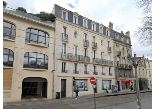
Fig. 12 The plot on 29 - 33, Cours Evrard de Fayolle, in Bordeaux, after the 2016 development [source: https://www.google.com/maps , retrieved October 7, 2024]
