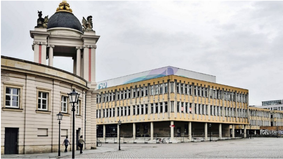
Fig. 7 The west side of the Old Market Square, in Potsdam, with the building of the Institute for Teacher Training, before its demolition in 2018 [source: Anker, J. (2017), from imago/Jürgen Ritter]
