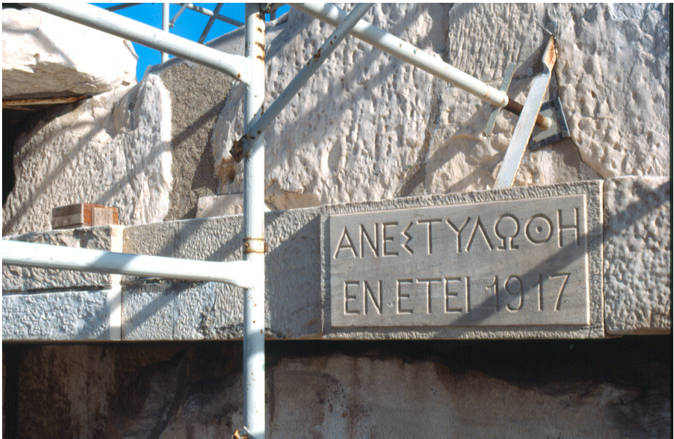
Fig. 3, 4. Athens, Acropolis. Restoration tiles in Pentelic marble, worked in a different way from the original, and with the date of restoration (1901, photo at the top, and 1917, photo at the bottom) inscribed, guaranteeing the distinctiveness of the authenticity of the original material. Author: S. Gizzi, 1994
