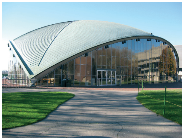
Fot. 1. Kresge Auditorium (1950–1955) Massachusetts Institute of Technology, Cambridge MA, Eero Saarinen (fot. M. Czarnecki 2007)
