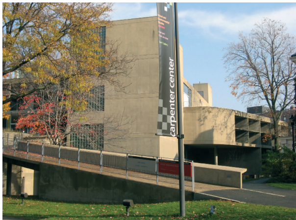
Fot. 2. Carpenter Center for Creative Arts, Cambridge MA, 1963, Le Corbusier (fot. M. Czarnecki 2007)
