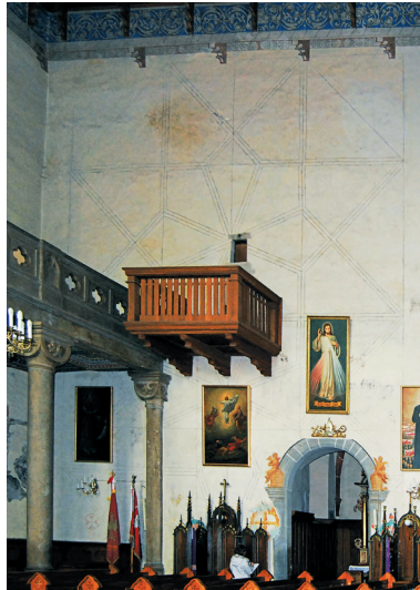
7. Szydłowiec, the design vaults on the wall of the north nave. Photo: J. Lewicki, 2016.
