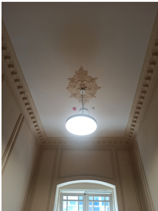
Fig. 9. Thessaloniki State Conservatoire, view of a typical ground-floor ceiling, with decorative plasterwork. Photo: Author
