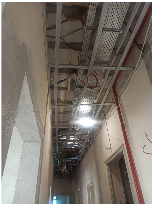
Fig. 10. Thessaloniki State Conservatoire, view of a typical, conventional first-floor ceiling, allowing concealment of equipment in a suspended ceiling. Photo: Author
