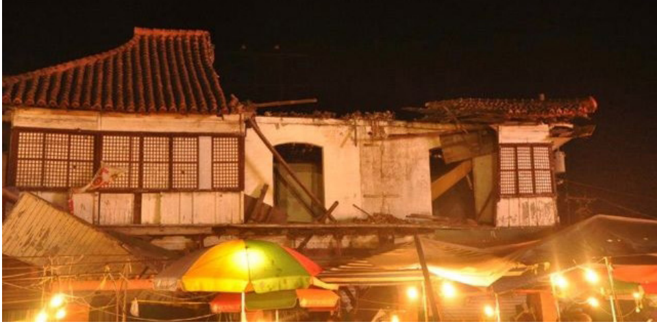
Fig. 4. The collapse of the original structure following systemic gutting of its interior components (Burningbatsu, 2012)
