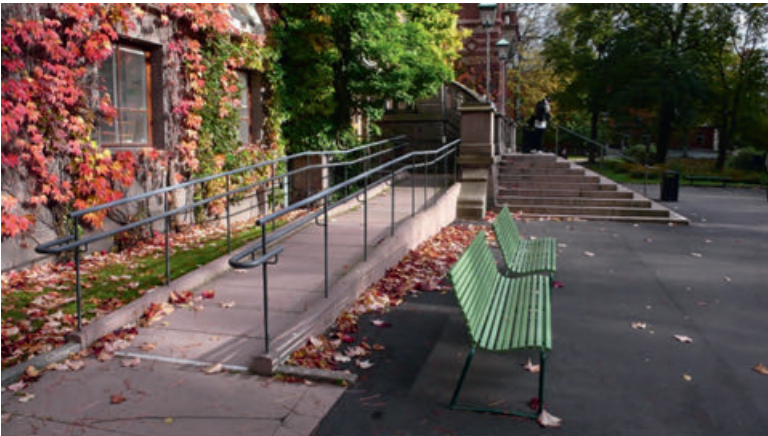
Figs 1-2. Lund (Sweden). Real effort was made so that the conservation of historical buildings could meet accessibility criteria. The station, the main building of the University, and its library constitute the best examples of such integration.
