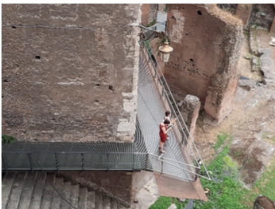
Fig. 37. Footbridge in Mercati di Traiano, Rome, Italy.
