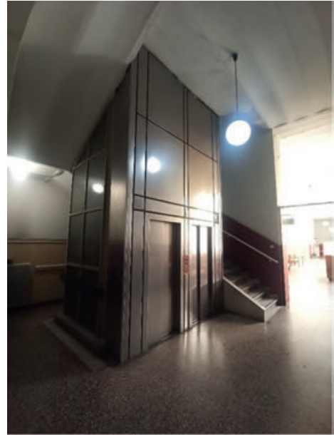
Fig. 23. Former Administration Building.
