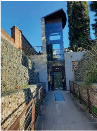
Fig. 30. New lift in Imperial Fora, Rome, Italy.
