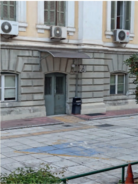
Fig. 12. Former Administration Building.
