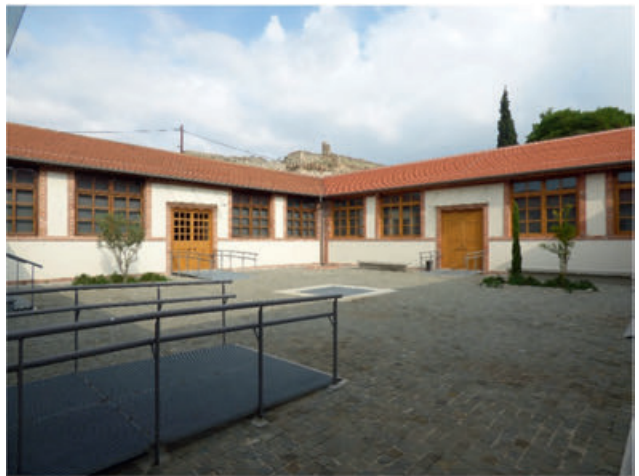
Fig. 19. The former Technical School “Hamidie – Islahane.”
