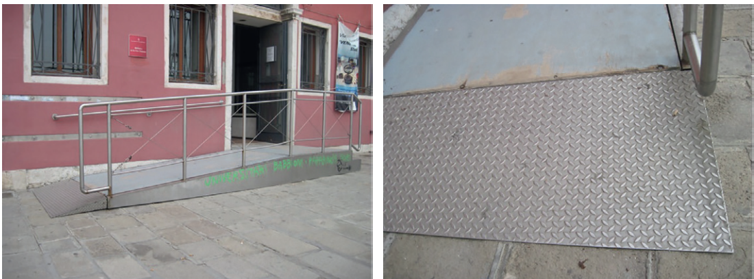
Fig. 13. Access to the building entrance with a ramp (with handrails) with a solid, corrugated and smooth running surface; Venice, Italy (photo by K. Kaperczak).
