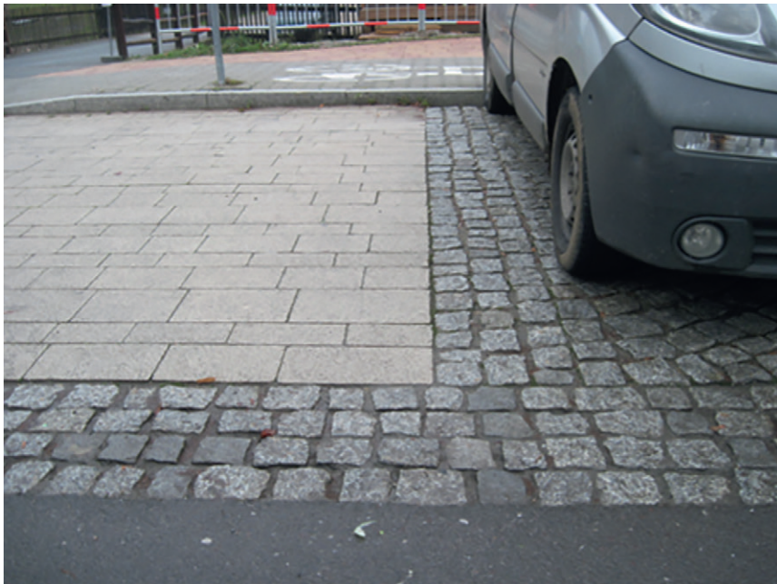
Fig. 6. Changing the pavement of a parking space for the disabled from split paving sett to smooth paving sett in Zakopane, Poland (photo by K. Kaperczak).
