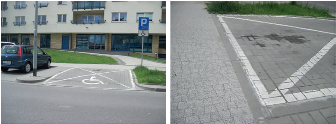
Fig. 8. Parking spaces made at the level of the adjacent sidewalk do not require overcoming height differences (faults) when accessing vehicles; Warsaw, Poland (photo by K. Kaperczak).
