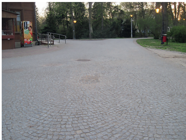
Fig. 4. Sidewalk pavement made of split paving sett hinders the movement of pedestrians; Ciechocinek, Poland (photo by K. Kaperczak).
