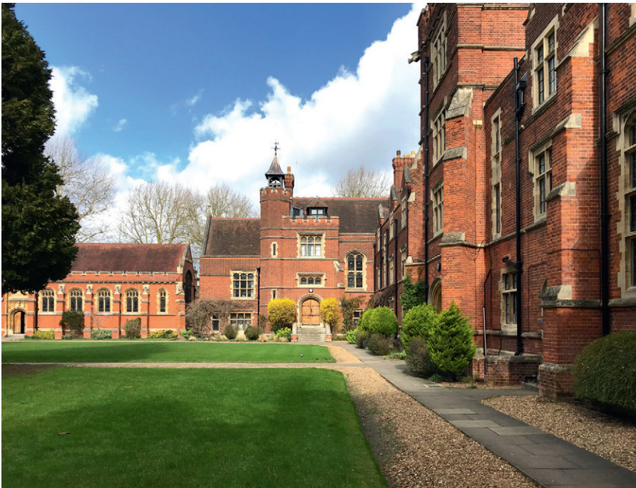
Fig. 1. Ridley Hall, Cambridge – east range, before the project.
