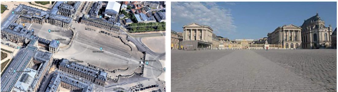
Fig. 2. View of the palace courtyards; after Google Maps (left). A strip of leveled pavement on the palace axis (right); photo by D. Sikora, 2018.
