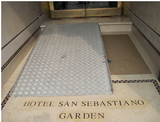
Fig. 12. Access to the building entrance with a ramp (without handrails) with a solid, corrugated running surface; Venice, Italy (photo by K. Kaperczak).
