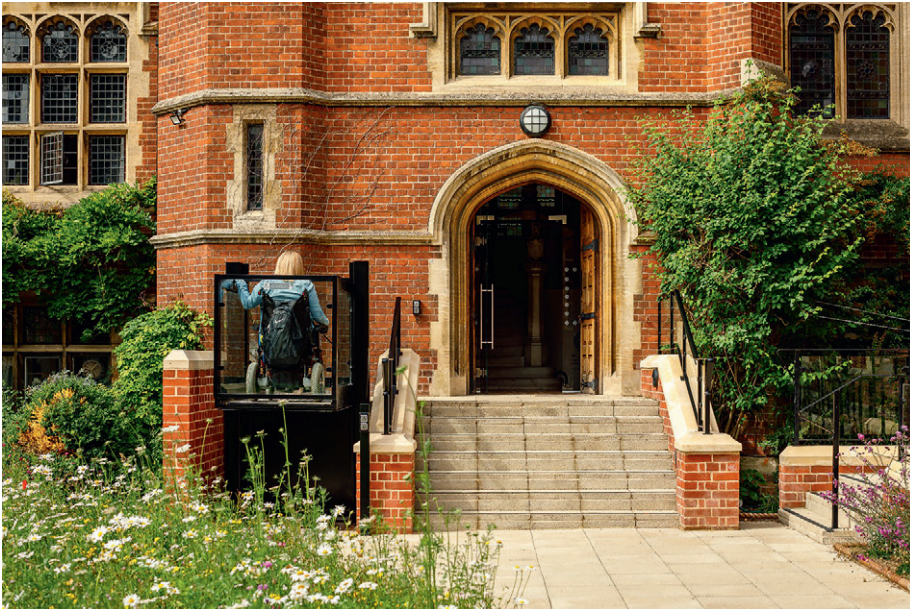
Fig. 2. Ridley Hall, Cambridge – Stair D, completed (photo: Lina and Tom Ltd).
