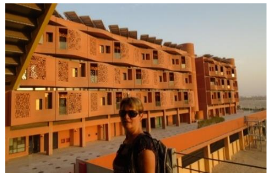
Photo 8. Solar panels on building roofs (photo by T. Niedzielska)
