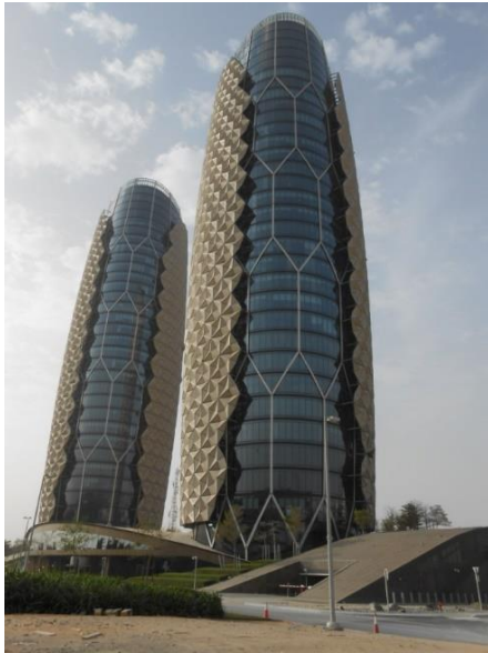
Photo 6. Al Bahr Towers. A view of the buildings from the north (photo by W. Sobczyk)
