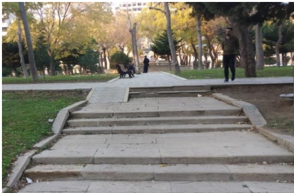
Figure 5. A ramp just in a staircase march in Officer's Park, Baku, Azerbaijan
