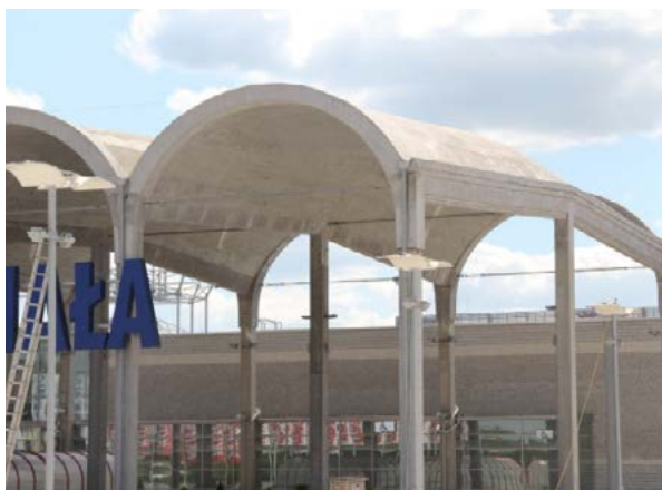
Fig. 19. Reinforced concrete vaults on the car park of the Biala Centre. Source: photograph of the authors, 2011
