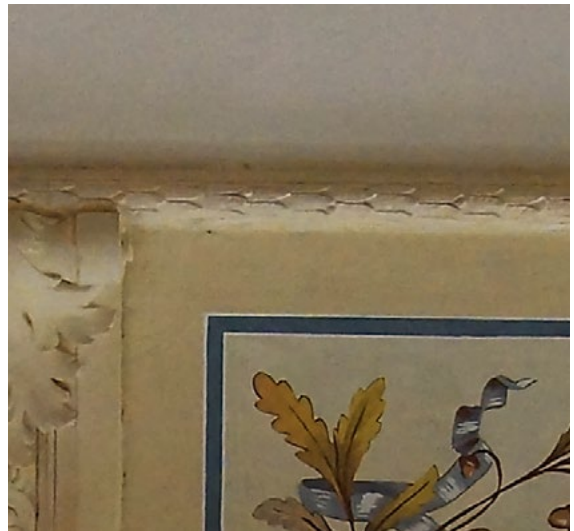
Fig. 8. The same fragment of the vault' surface of the molded decorations after the conservation, 2015. Photo by S. Hetmanchuk.
