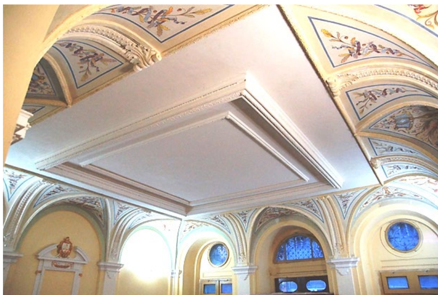
Fig. 17. The main lobby of the 19 th academic building of L'viv Polytechnic National University in 2015 after the completion of reconstruction and restoration works (photo by M. Bevz).
