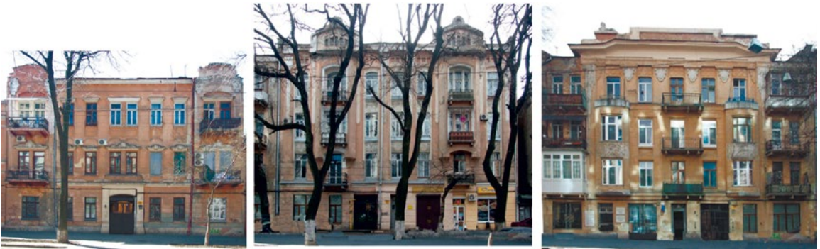
Fig. 2. Russov's Revenue Houses, architect: L.M. Chernigov, early 20 th century, the facades
