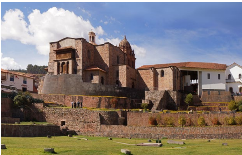
Fig. 5. The curved wall of the 'balcony' of the Coricancha (photo Jacek Kościuk).
