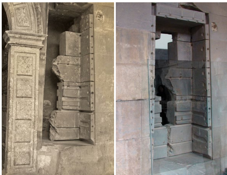
Fig. 4. Coricancha. The niche in the facade of the „Room of the Stars”. Left: situation by 1942. (Photo from the John H. Rowe private archive – courtesy Patricia J. Lyon). Right: the present day view after reconstruction by Oscar Ladrón de Guevara. (Photo Jacek Kościuk).
