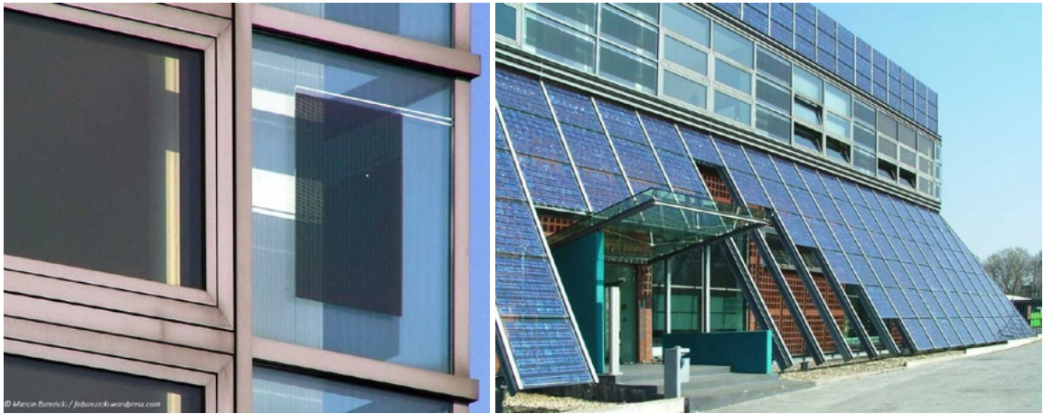
Fig. 9. Homogeneous systems thin-film semitransparent module in insulating glazing applied in the visible part of the window. Photographs by M. Muszyńska-Łanowy.
