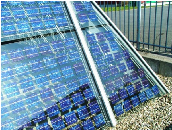
Fig. 4. The example of the use of dummy glass-glass module. Cell in trapezoid module visible of the figure are not connected to the grid. (Optisol®, manufactured by Scheuten) – photographs by M. Muszyńska-Łanowy.
