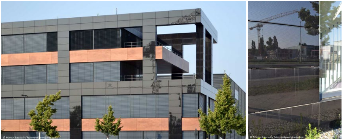
Fig. 3. Black Copper Indium Gallium Selenide (CIGS) cells used on the façade of the Solteure Headquarters, Berlin-Adlershof (arch. Rainer Girke, 2009) – photographs by M. Muszyńska-Łanowy.
