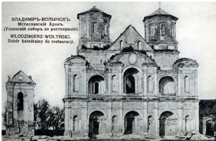
Fig. 3. West elevation of the Cathedral of Dormition. Postcard. End of 19 th cent.
