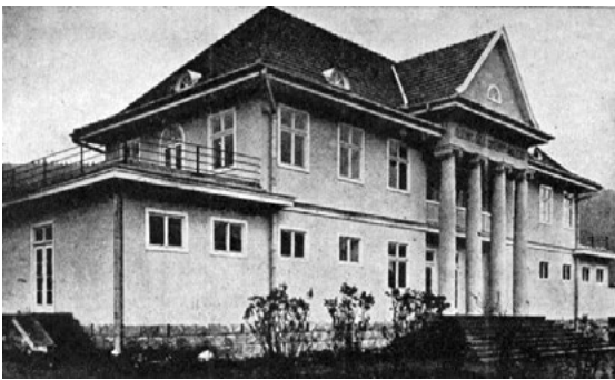
Fig. 1. Jaremzcze. Bathing facility of dr Józef Matuszewski. Design: Max Zucker, 1935. Postcard from 1930s from the author's collection
