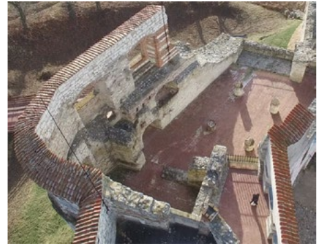
Fig. 7. Photo 4 Shaping the crown of the wall
