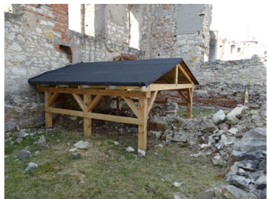
Fig. 9. Photo 6 Shaping the crown of the wall
