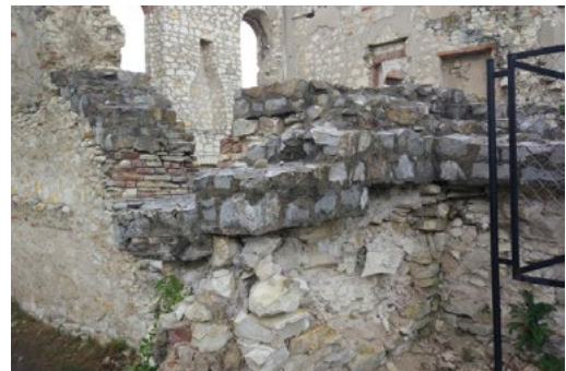
Fig. 3. Photo 2 Bricklaying the crown of the wall with a quartzite stone
