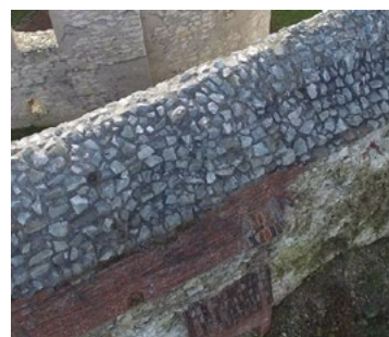
Fig. 5. Photo 3 Shaping the crown of the wall
