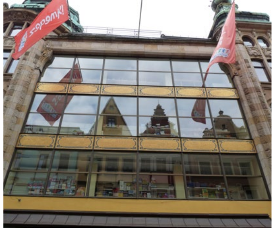
Fig. 12. Close-up look at the facade of Feniks Department Store building refurbished in accordance with the design of Kirschke Pracownia Projektowa (photo by P. Kirschke).
