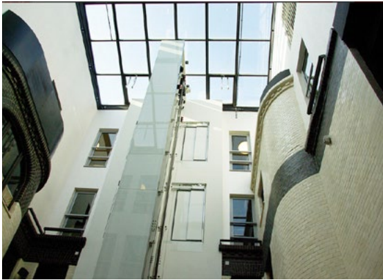
Fig. 20. The multi-story atrium of Hieronimus I Office Building refurbished in accordance with the design by Grupa 33_03 – a view showing the new glazed elevator shaft (photo by Grupa 33_03).
