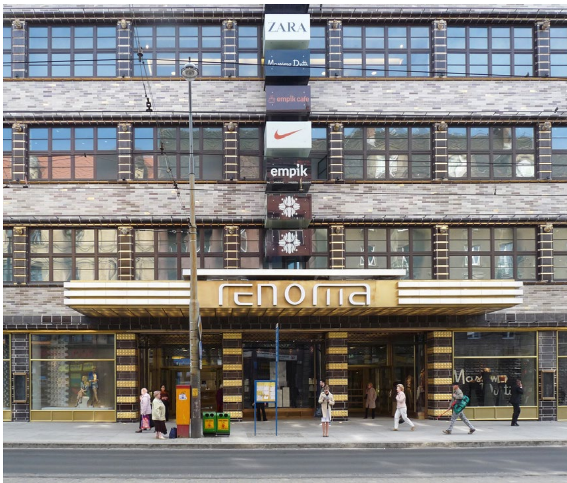
Fig. 5. The main entrance to Renoma Department Store, refurbished and extended in 2005–2009 in accordance with the design of Pracownia Projektowa Maćków (photo by P. Kirschke).
