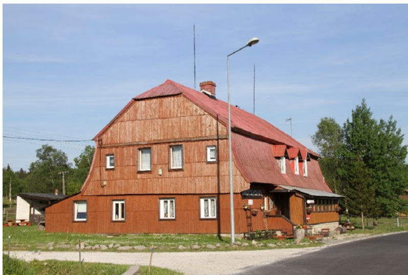
Fig. 25. Lasówka. An agritourism building, Chata Sudecka , with distinct regional features. Particularly noteworthy is the huge mansard roof, which houses a freely living story. Construction – early 20 th century. Such buildings can be found in other locations in the Kłodzko Land and on the Czech side of the border. Photo by the author – 2017.
