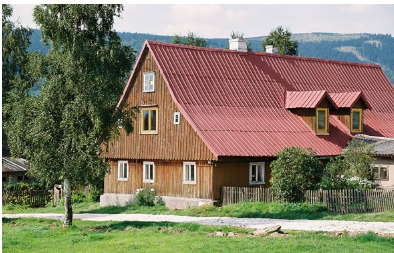
Fig. 17. Lasówka. The former Erlitztalbaude hostel* near Mostowy Potok . Visible regional features of the building's architecture. Currently a private property. Photo by the author – 2005.
