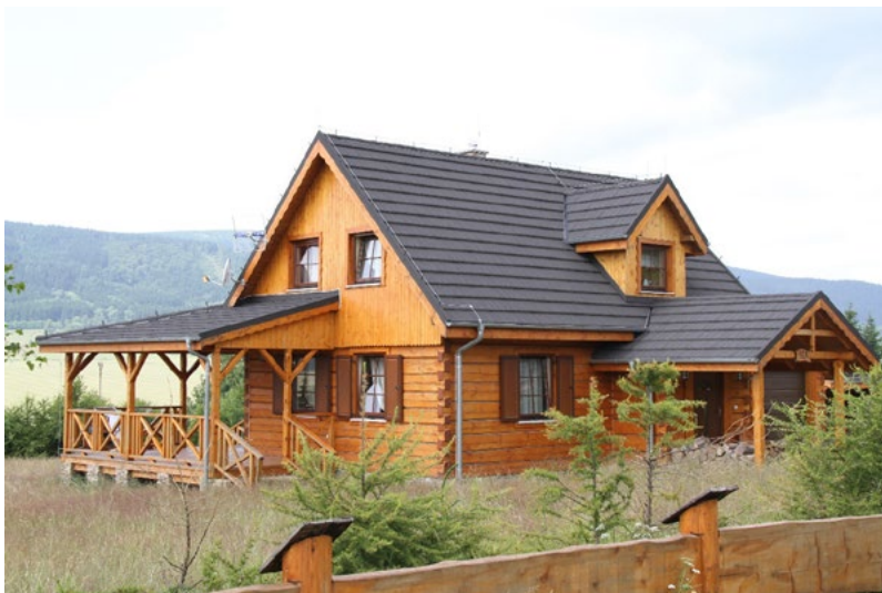
Fig. 23. Lasówka. A holiday home built in 2010. Photo by the author. 2014. It is a pity that despite the wooden construction of the building and quite careful workmanship, there is a lack of regional identifiers of architecture of the Kłodzko Land.
