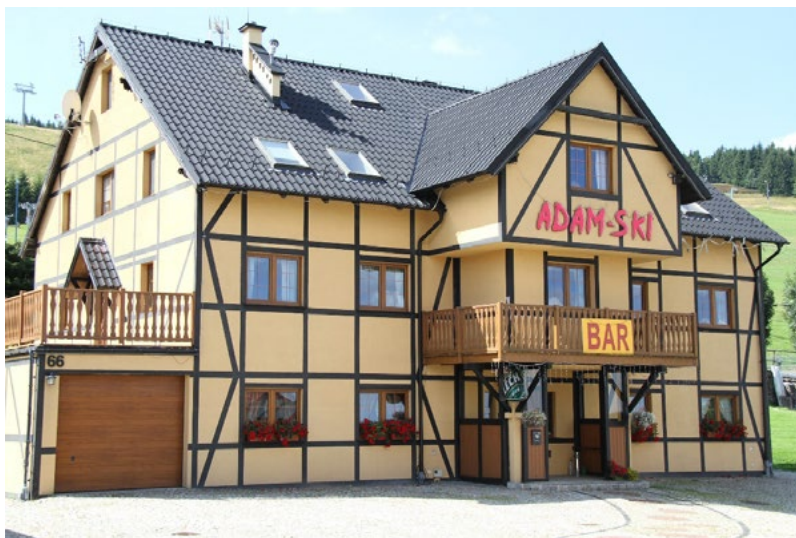
Fig. 11. An unprofessionally designed arrangement of transom structure elements on the walls of the ground floor and the first floor of the hotel building in Zieleniec, designed to suggest a real structure, gives the impression of artificiality and randomness to an outside observer.
