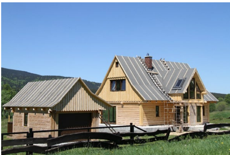
Fig. 24. Lasówka. A single-family building with a wooden structure and a garage under construction. It is a relatively successful attempt to refer in the architecture of the building to the regional heritage of the Kłodzko Land. Photo by the author. 2017.
