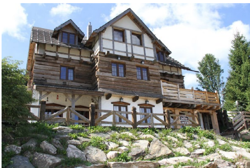
Fig. 10. A recently constructed guesthouse in Zieleniec with quite surprising structural and formal solutions of external walls. The transom system of attic beams contrasts with the wooden and log load-bearing system of the first floor (recycled building material), and brick walls (?) of the ground floor. Photo by the author – 2017.
