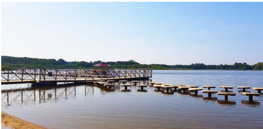
Fig. 3. Osieczna – Contemporary pier and walking path of circles (photograph taken 15.09.2020 by the author).
