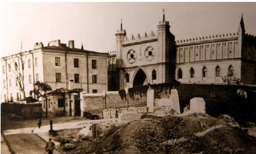
Fig. 7. Administration building, museumlubelskie.pl , access 2019.
