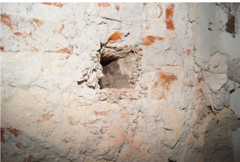
Fig. 8. Wooden box/channel cut in the external wall of a building, photo: K. Janus, 2016.
