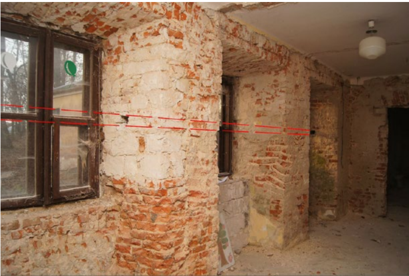
Fig. 7. Location of a canal/ wooden box cut with secondary windows, photo K. Janus, 2016.
