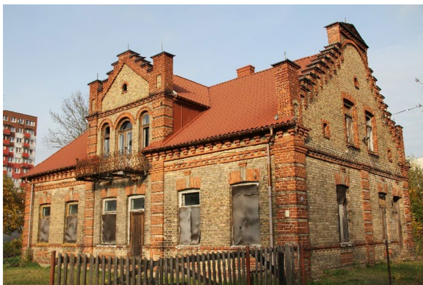
Fig. 4. House at Grunwaldzka Street – the present state (on the right). Photo: Andrzej Tokajuk
