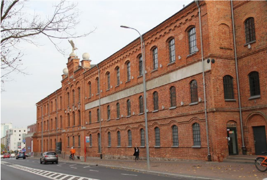
Fig. 1. The Mercury building from the factory complex of the Eugeniusz Becker Society of Białystok Manufacture at Świętojańska Street – the current state. Photo: Andrzej Tokajuk
