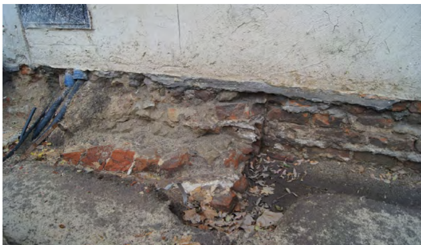
Fig. 8. Wall discovered in the excavation of the northern sacristy wall
