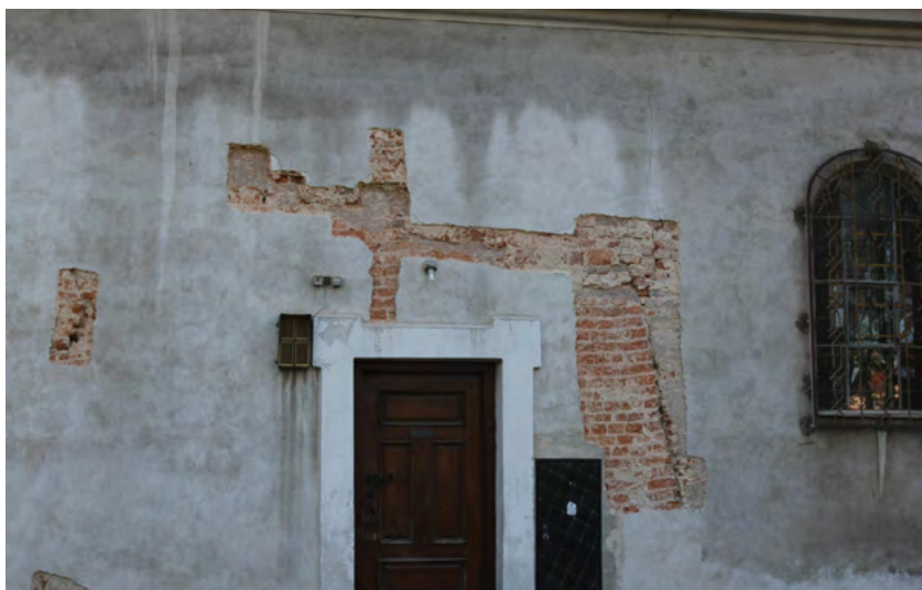
Fig. 6. Uncovered buttress edge of the northern sacristy wall
