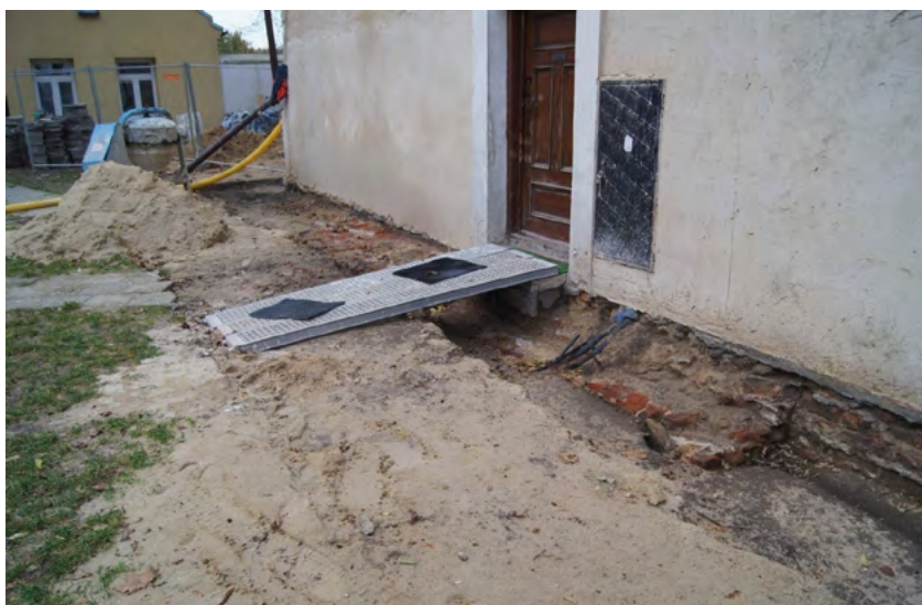
Fig. 7. Wall discovered in the excavation of the northern sacristy wall
