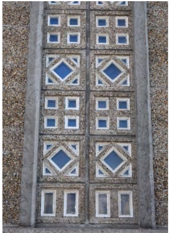
Fig. 6. Detail on the façade of the church – visible stained glass windows, concrete bands and the structure of the wall. Source: Szumigala K.O.
