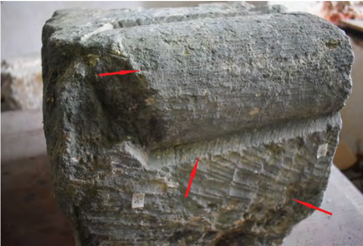
Fig. 11. Detail from glauconite (the corner stone block with a half column) with marked traces of handling (photo M. Bevz).
