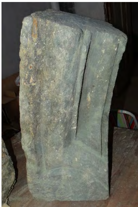
Fig. 18. Profiled block of glauconite. Probably an element of the portal arc. Photo by M. Bezv
