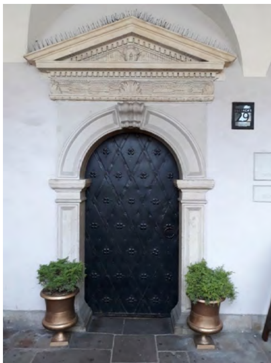
Fig. 5. Portal, Staszica 29, author's photograph
