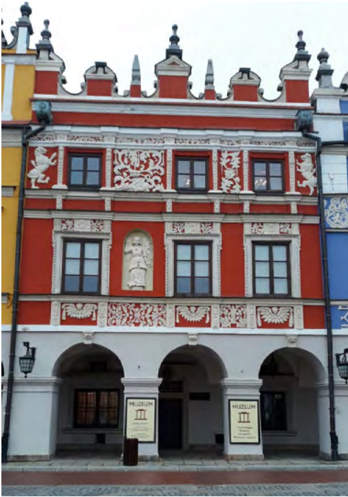
Fig. 6. The tenement house, the Bartoszewicz Family – owned (till the end of 17 th c.) 1 , the so-called “under the Archangel Gabriel”, “under the Lions”, one of the Armenian houses, north façade of the Great Market Square, the headquarters of the Zamość Museum, author’s photograph
