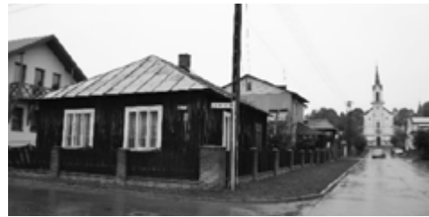
Fig. 5. Market square buildings and the church at the close of the North-South axis (photo by Sosnowska)
