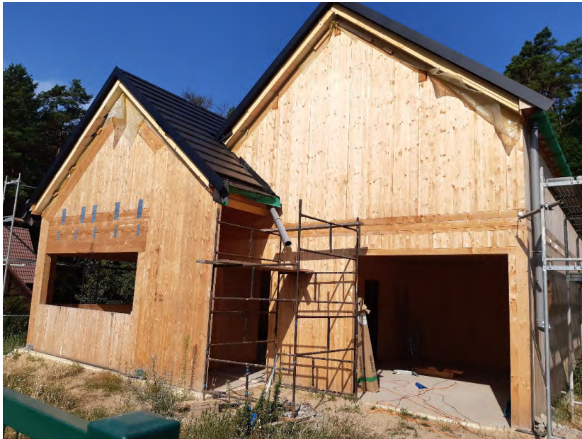
Fig. 2. Building in a wooden structure. Own photo
