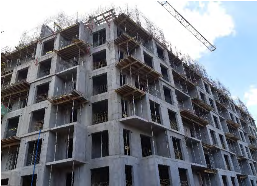
Fig. 1. Reinforced concrete structure. Own photo
