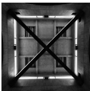
Fig. 9. The central void's roofing, 2010.
