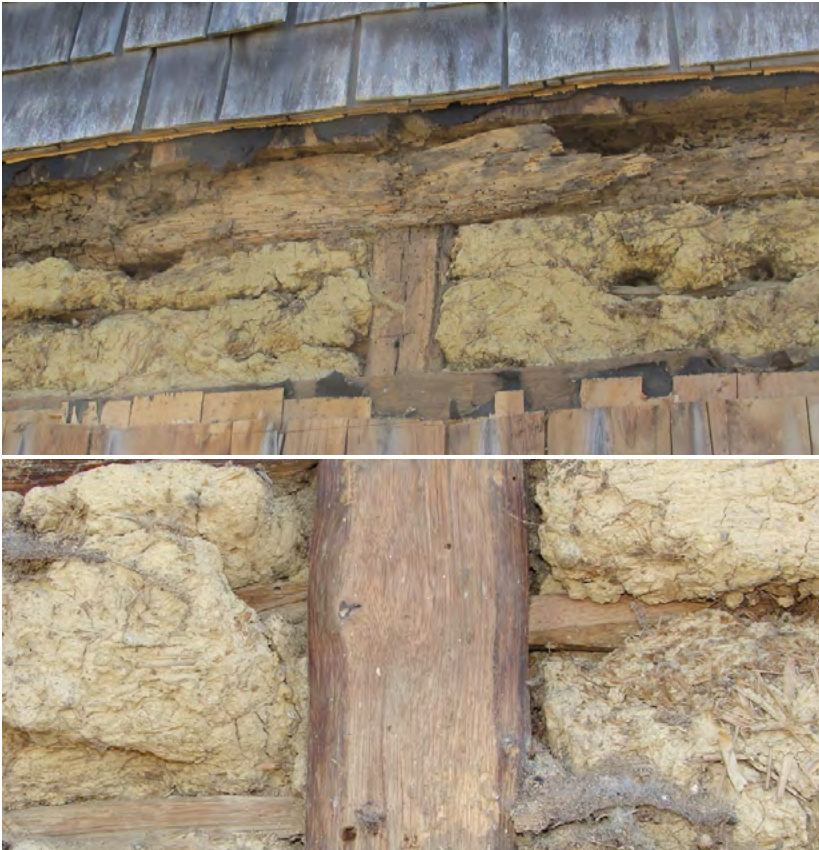
Fig. 5. Top: Clay and straw infill in the exterior wall of the Hancock-Mitchell House, Chilmark, Massachusetts (Myron O. Stachiw, 2015)
