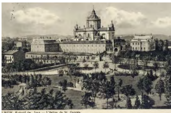
Fig. 7. St. George Monastery Complex [4]
