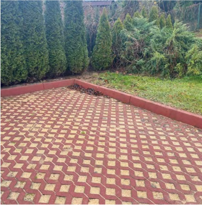
Fig. 5. Existing surface of the car park. Source: Own photo
