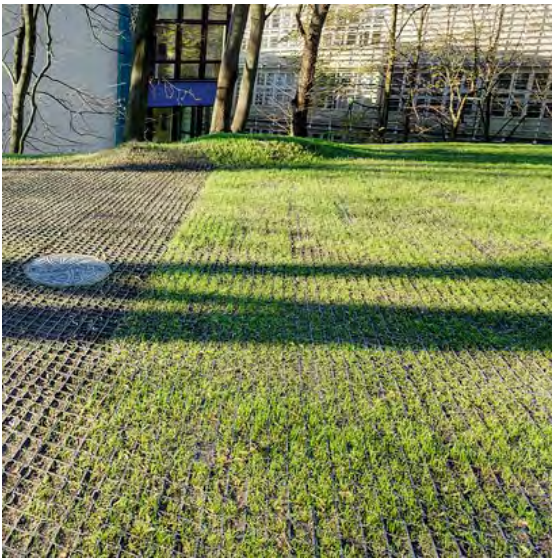
Fig. 8. Example of geogrid usage. Source: www.geoproduct.pl
