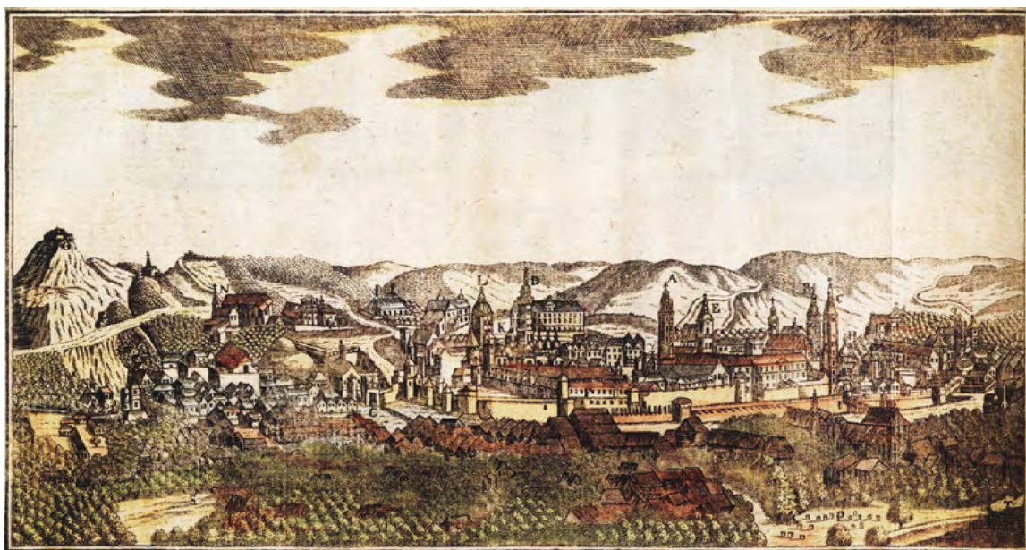
Fig. 2. Panorama of the Old (on the left) and New Midtown areas of Lviv on an engraving by Georg Borovsky from the late 18 th century (M. Kapral "Lviv. Atlas..." [1])
