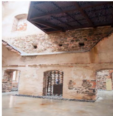
Fig. 26. Openwork door made of corten, 2022, by K. Drobek
