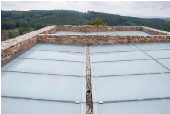
Fig. 12. Glass roof hidden below the wall topping line, 2022, by K. Drobek
