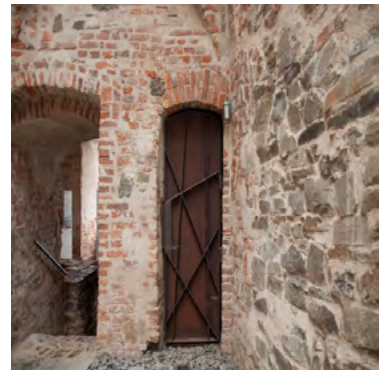
Fig. 27. Solid doors made of corten, 2022, by K. Drobek
