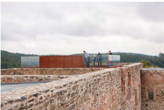
Fig. 14. Large panoramic terrace with balustrades made from corten and glass, 2022, by K. Drobek
