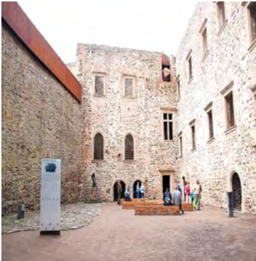
Fig. 16. Information board and outdoor lamp located in the courtyard area, 2022, by K. Drobek
