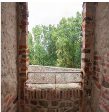
Fig. 19. Guard rail at window opening, 2022, by K. Drobek
