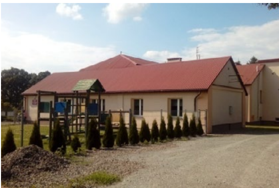
Fig. 3. Building of the Elementary School (by M. Stefanek, 2017)
