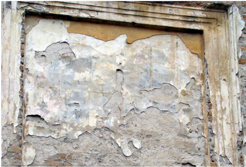
Fig. 20. Photo of the remains of artistic fictional paintings (the window) on a wall of the castle in Zhovkva. Photo by M. Bevz, 2012.
