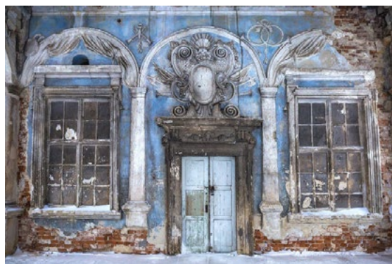
Fig. 18. Photo of stucco and painted fictitious windows on the eastern terrace of the castle in Pidhirtsi (present state). Photo by E. Shavlovskya [12].
