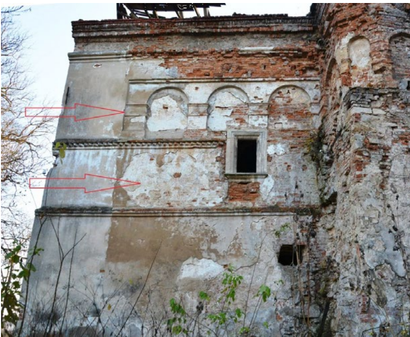
Fig. 3. The north wall of the corner tower of the Pomoriany castle. The places where the polychrome paintings preserved are indicated with arrows. Photo by M. Bevz, 2017.
