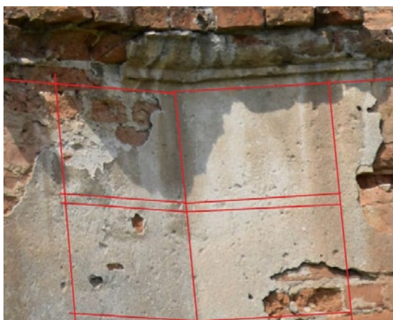
Fig. 23. The fragment of the outer wall of the west wall of the Stare Selo castle. The lines indicate the marking on the plaster for painting. Photo by M. Bevz, 2019.
