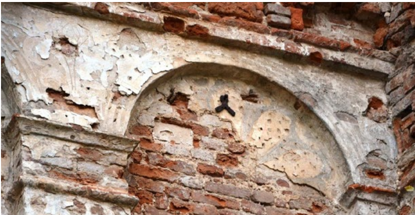
Fig. 6. Hand circle-drawn archivolts and half-rosettes in the arch belt on the 3 rd tier of the outer wall of the tower. On the left side to the arch are fragments of a rose with branches. Photo by M. Bevz, 2017.
