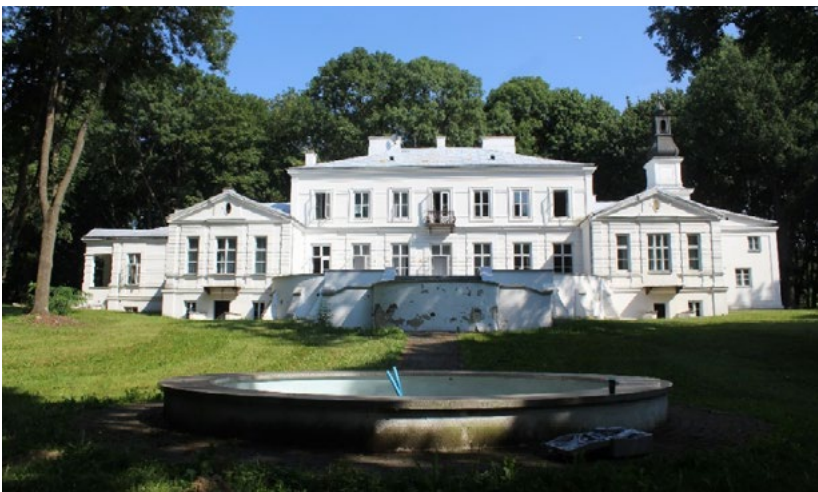
Fig. 2. South façade. (author's own photograph)
