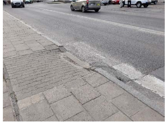
Fig. 14. Limited access to the zone of the pedestrian crossing, The Stefanidesa Square, Zamość. Photo: K. Kielin
