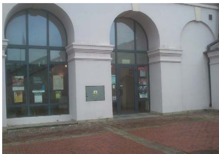
Fig. 6. The entrance to the Town Hall Customers' Office. Access provided by means of a small ramp, Zamość. Photo: Katarzyna Kielin
