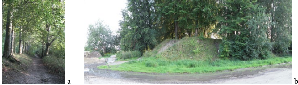
Fig. 3. A – The tree stand forming an alley on the embankment crown, B – A view at the beginning of the embankment from Chopina Street – differences in the levels and tree stand are visible. Source: The authors' photographs, summer 2012.
