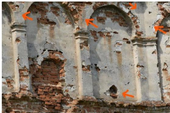
**Fig. 22.** The photo of the arcade belt of the upper part of the outer wall of the Stare Selo castle. Arrows indicate traces of marking for painting on plaster. Photo by M. Bevz, 2019.
