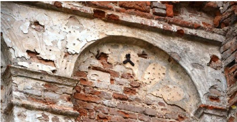
**Fig. 6.** Hand circle-drawn archivolts and half-rosettes in the arch belt on the 3<sup>rd</sup> tier of the outer wall of the tower. On the left side to the arch are fragments of a rose with branches. Photo by M. Bevz, 2017.
