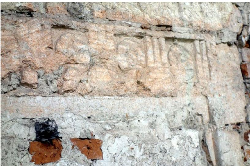
**Fig. 12.** Fragment of the south wall of the castle in Pomoriany. The carved window framing is made in limestone. The scenery is made up of carved rosettes and triglyphs arranged alternately. The carved forms were partially cut down during the rebuilding of the castle in the 17<sup>th</sup> century. Photo by M. Bevz, 2017.
