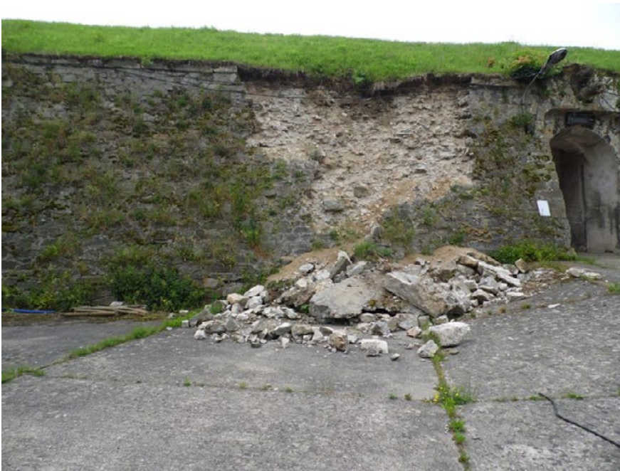
Fig. 3. Photograph showing the wall face (2018) – authors' own photograph
