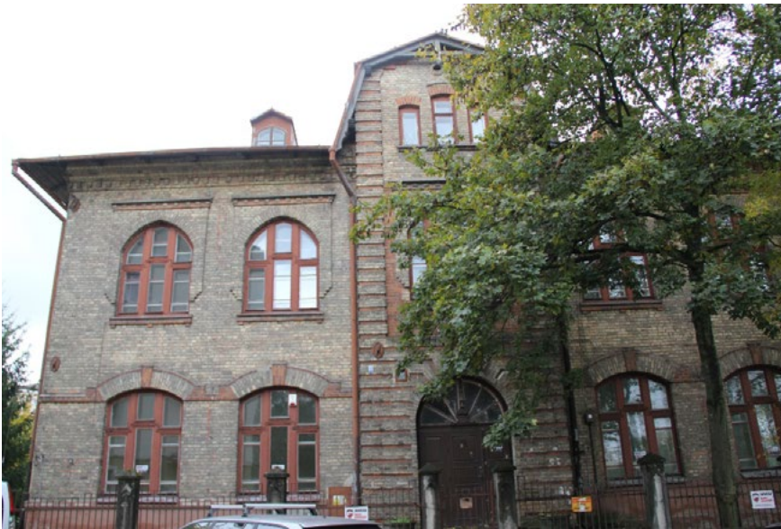
Fig. 5. Jewish religious school in the Talmud Tory school complex, Lipowa Street – the current state. The characteristic facade is made of two-color brick. Photo: Andrzej Tokajuk
