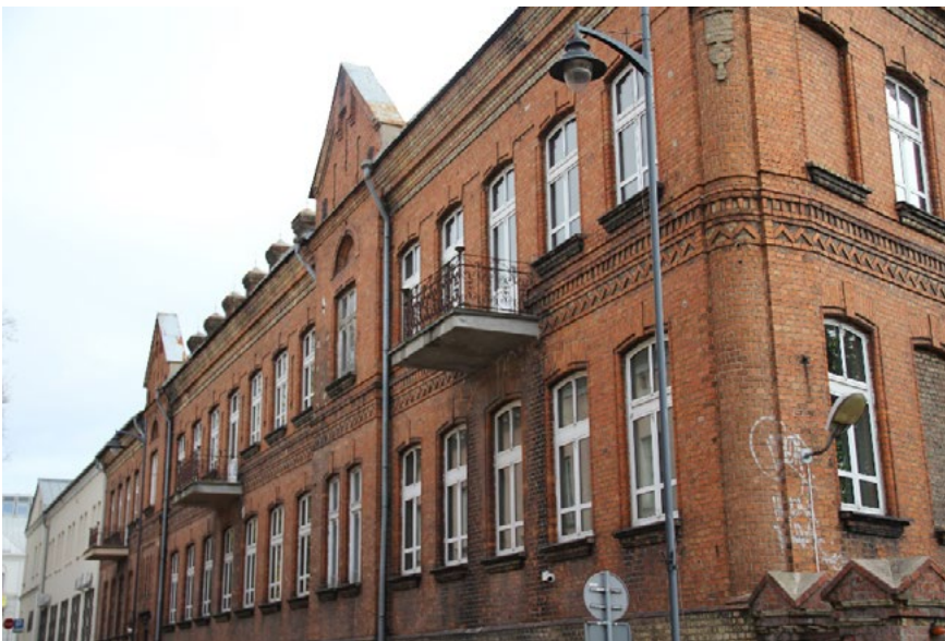
Fig. 2. The building of the former Juliusz Flaker textile factory (now a technical telecommunications building, Kościelna Street – two-story building represents outstanding architectural values, built of red brick, with the use of yellow brick only in the eaves cornice – present condition. Photo: Andrzej Tokajuk
